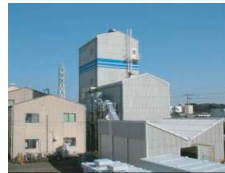
Appearance of the equipment building
