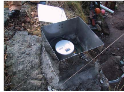
Strong-motion sensor installed on rock outcrop
